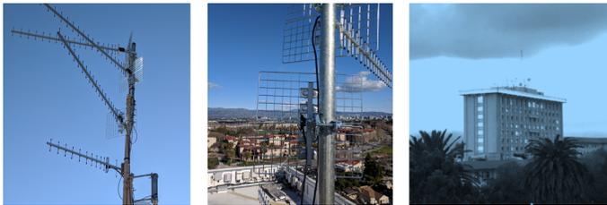
Fig. 4: Four directional antennas connected to the Gateway. The Gateway has been installed on top of a 11-level building in Santa Clara, California.
